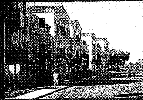
Phase 1 of Student Housing was completed in 2005, was fully occupied by its first residents, and should house in total 130 students by 2009 or 2010.
