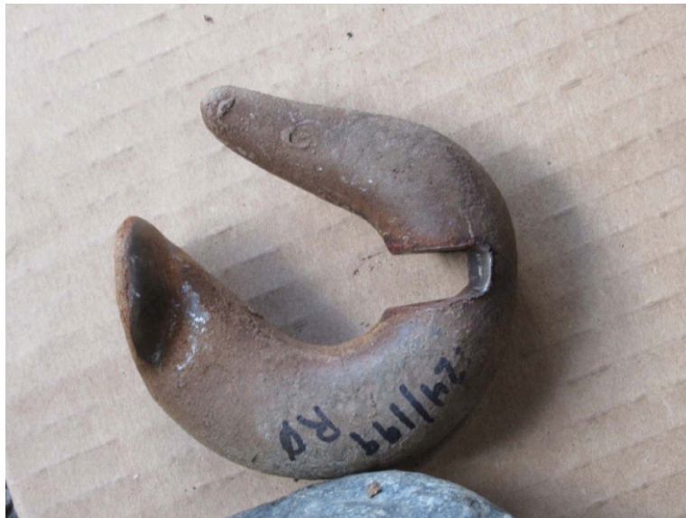
The deep gouging of a C-hook, caused by many decades of swaying in high wind (Dkt. No. 1123, Exh. A).
